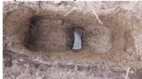
Inspection hole #2 post load test
