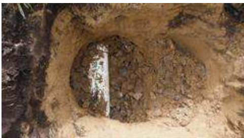
Inspection hole #1, clean material
