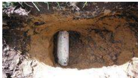
Inspection hole #2, clean material
